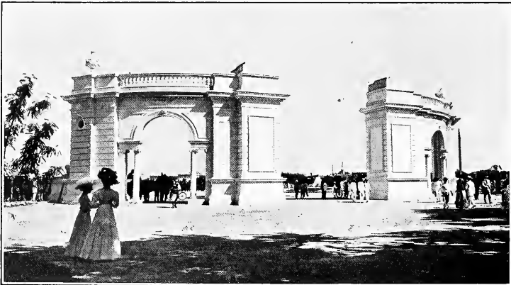
ARCH BUILT TO CELEBRATE THE CENTENNIAL, MERIDA.
